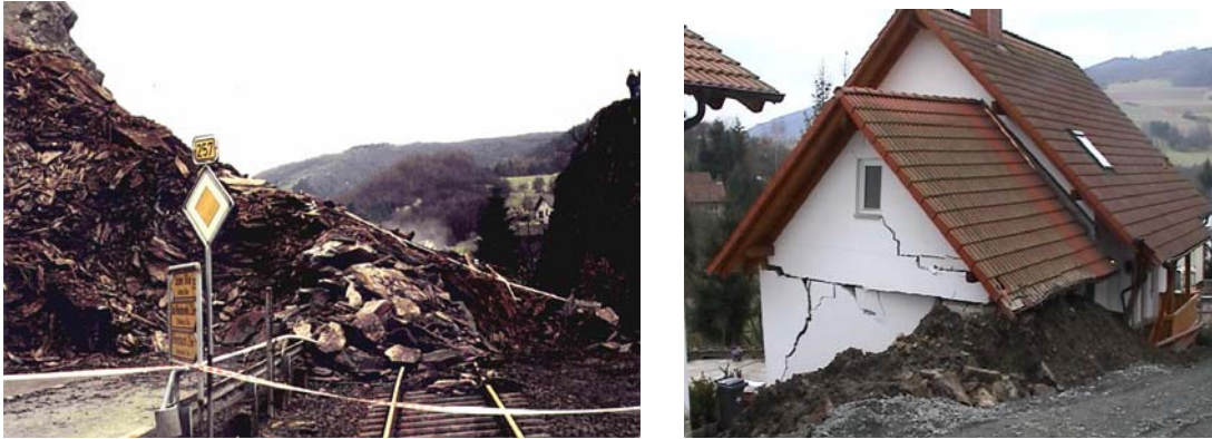
Figure 1. Blocking of a road and a railway line due to a rockfall and destroying of a residential building caused by a landslide
