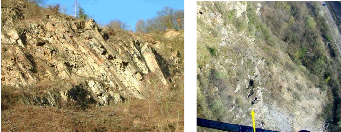
Figure 5. An apparent stabile 30 m high rock slope (on the left). Only the view from the helicopter shows the instability of the slope. Gaps (arrow) separate the front of the rock from the solid rock (on the right)
