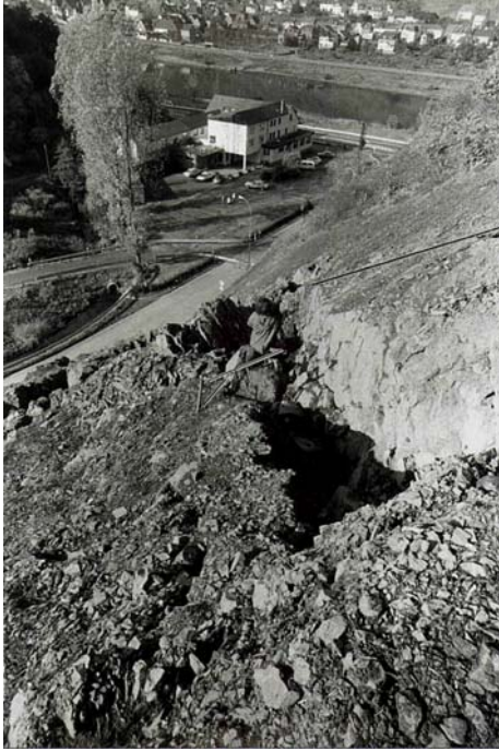
Figure 2. Opening of gaps on the rock slope
